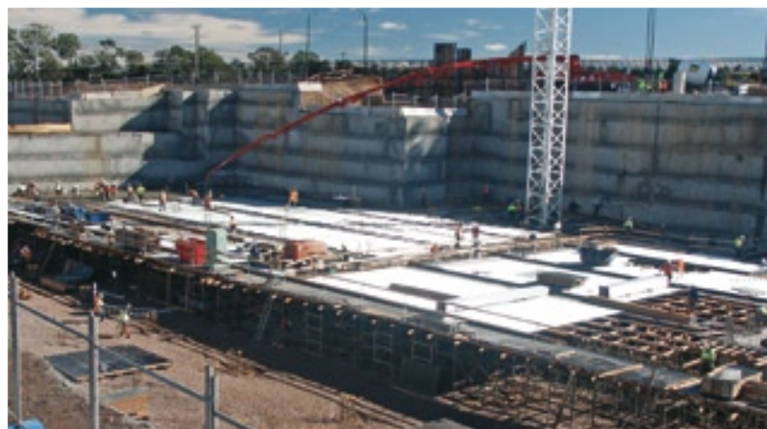
The deep basement required major excavation in rock
