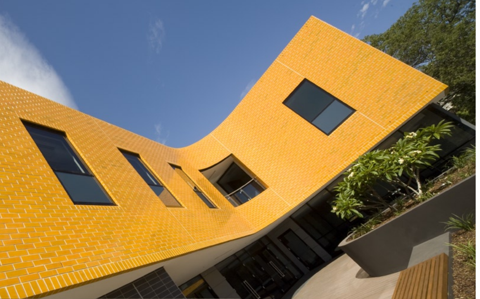
South facade showing complex shapes
