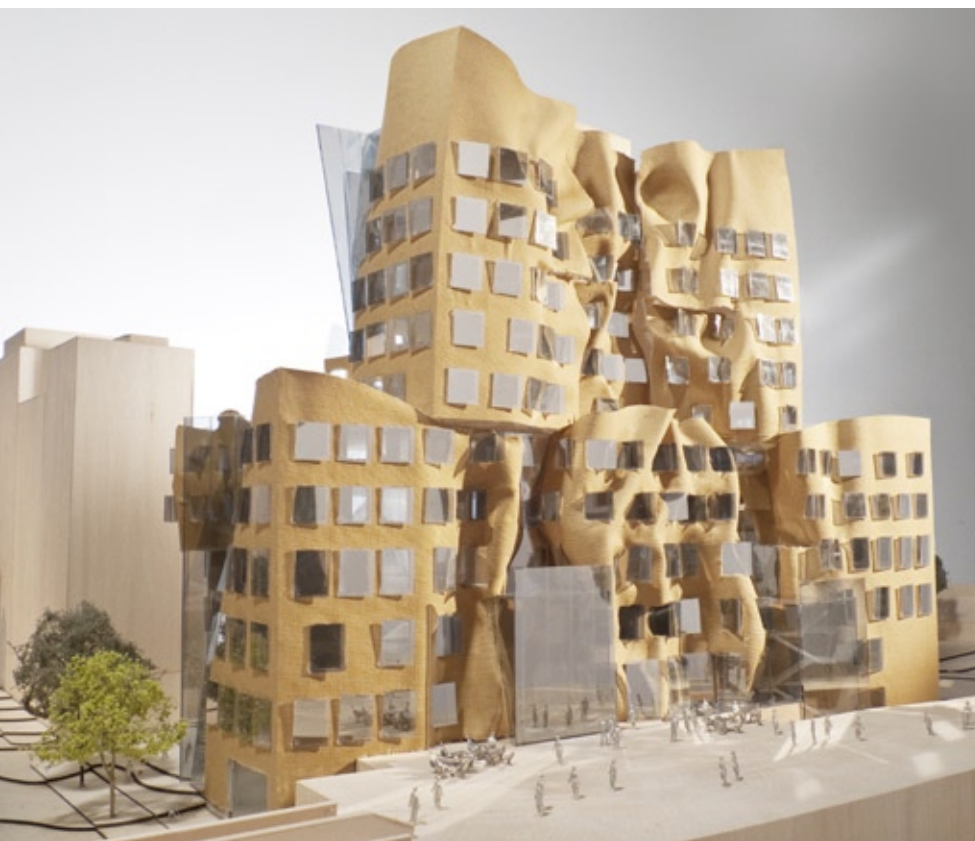
East façade, view across Ultimo Pedestrian Network, model scale: 1-to-100, photo courtesy of Gehry Partners
